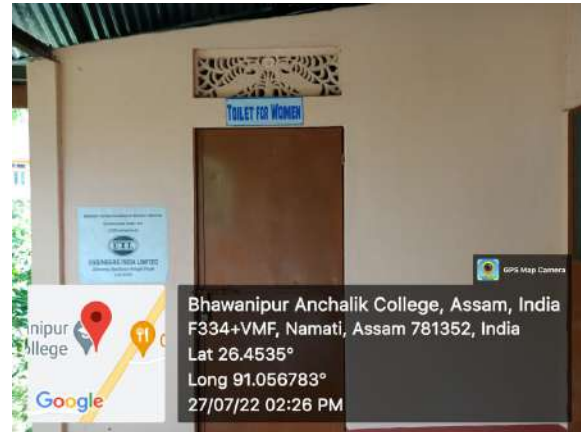
Women Toilet (Within Classroom Campus)
